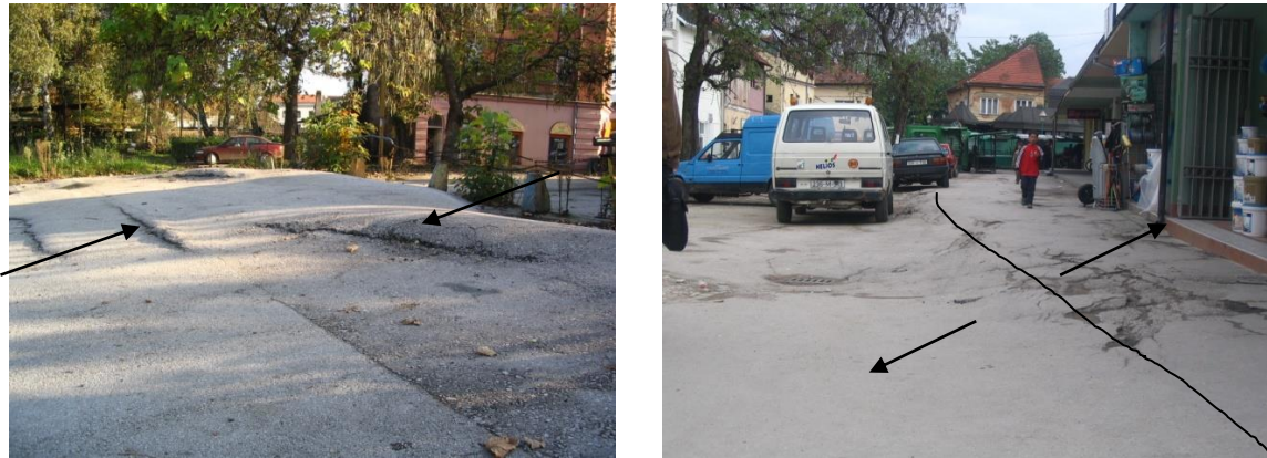
Figures 5.,6. Compression (left) and tension (right) deformations, salt mine (Tuzla, B&H) [4]
