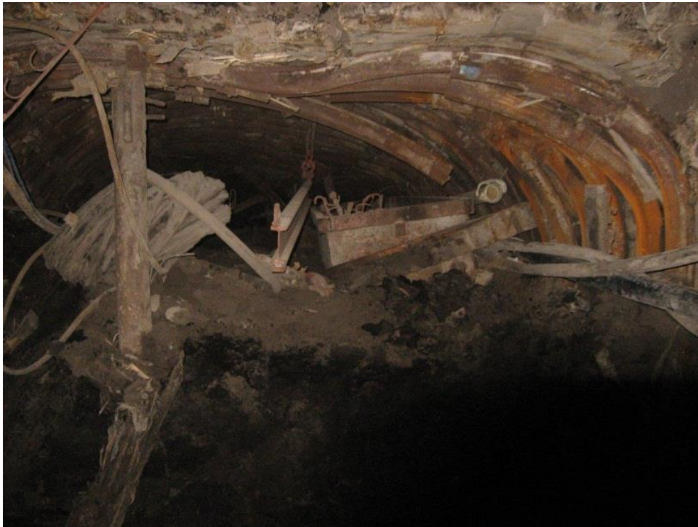
Figure 2: Consequences of the rock burst of 29 July 2014 in the former transverse conveyance line from G-panels at the height point k. -115.
